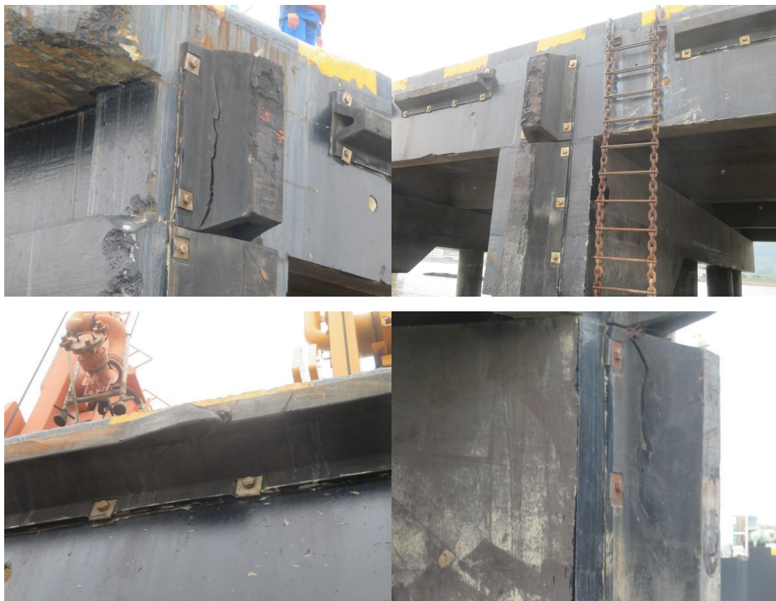
(1) 橡胶护舷开裂、破损
