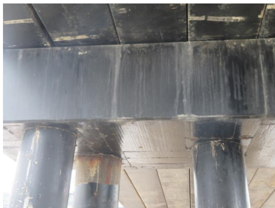
(1) 4-1#桩桩顶混凝土涂层脱落
