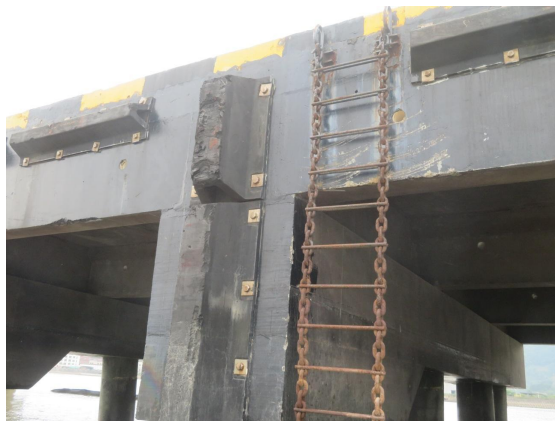
(1) 锚链爬梯锈蚀
